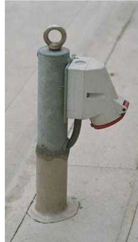
Weatherproof Power socket
